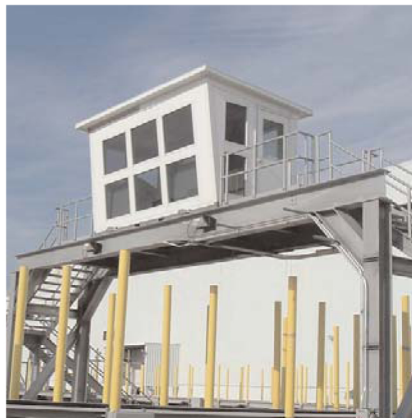
Crane-liftable tilt wall operator booth with a 130 mph wind load rating.
