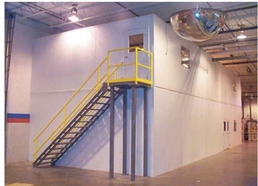
3. 2nd story completed with stair system access.
