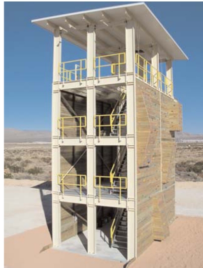
A four story air-attack training tower
