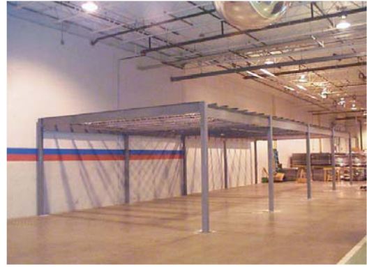
1. Build a mezzanine.
